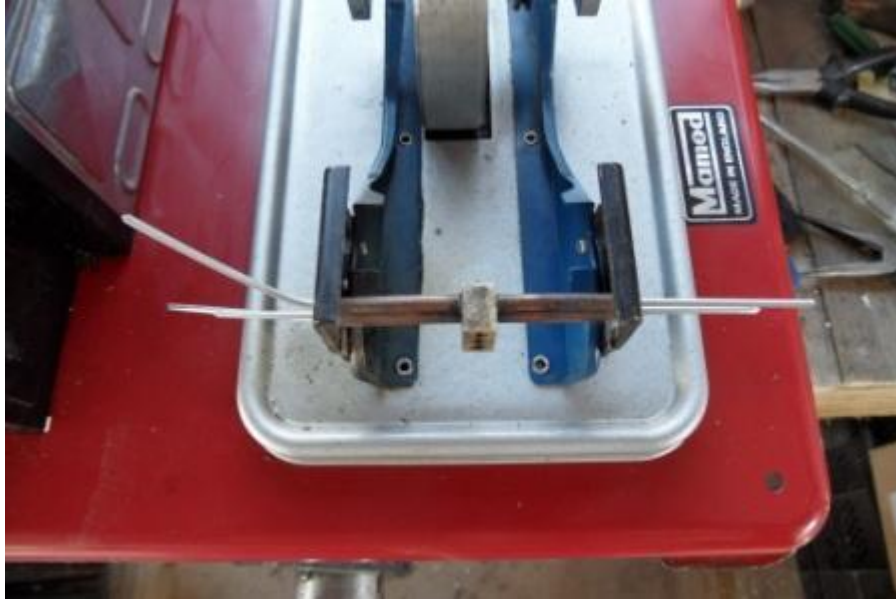
Multiple rodding of pipes prior to soldering
