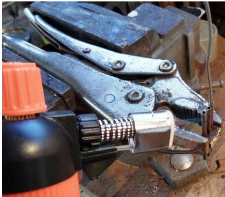
Removing hard solder from the pipes
